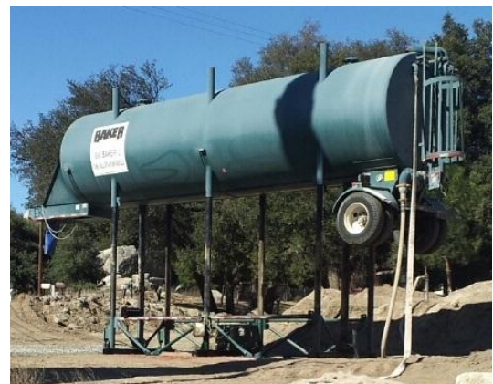
One storage tank by the pond
